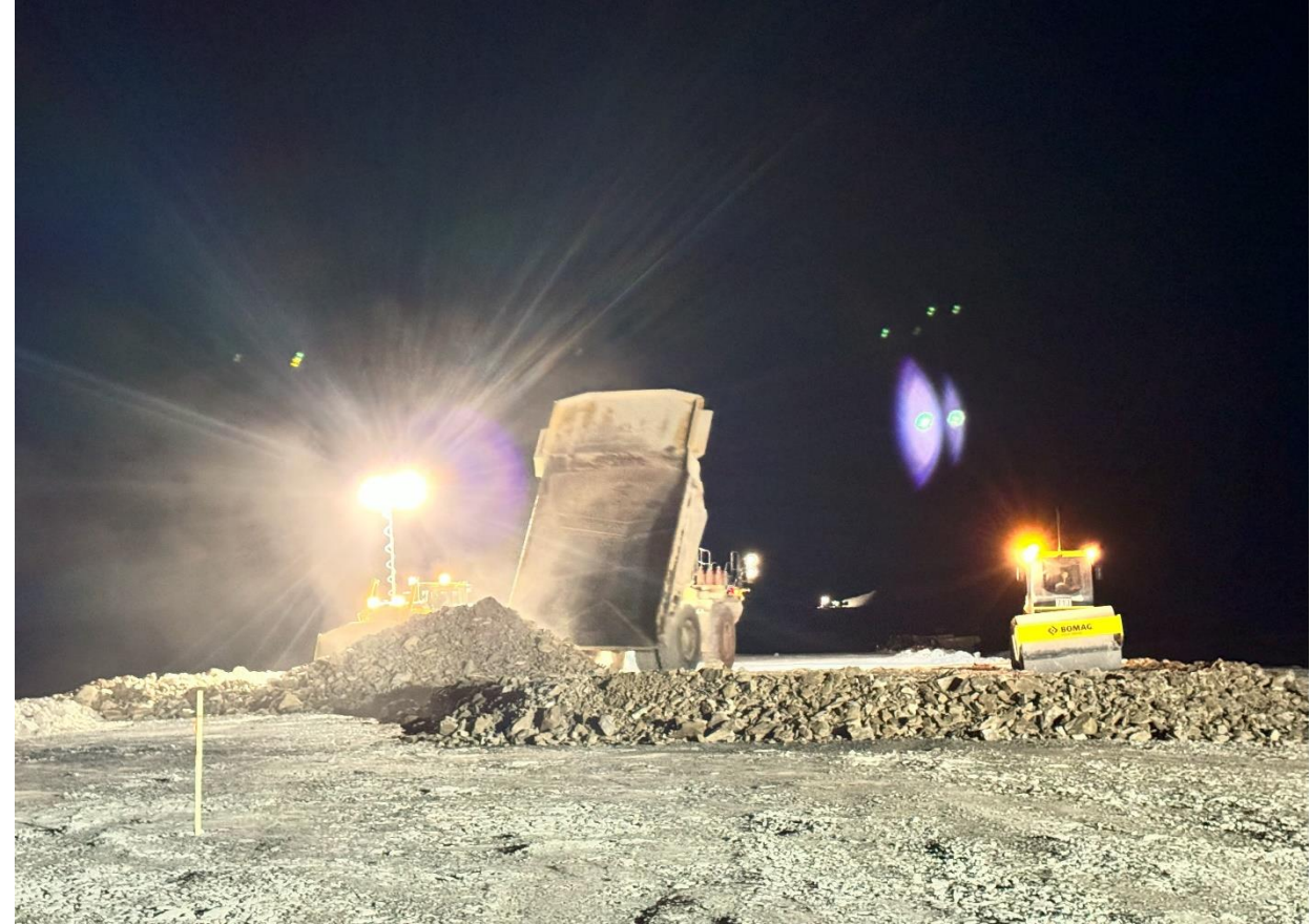
Tailing Management Facility Rock Placement
