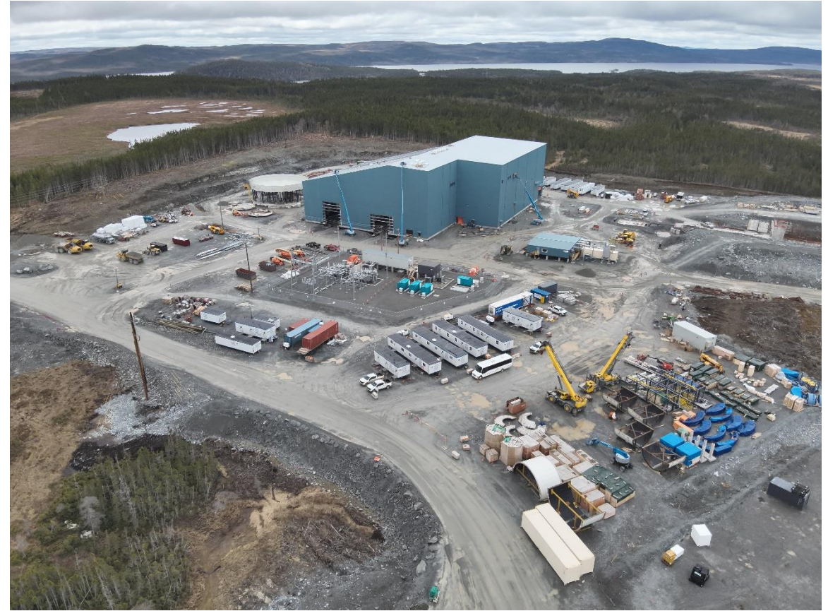
Process Plant Northeast
