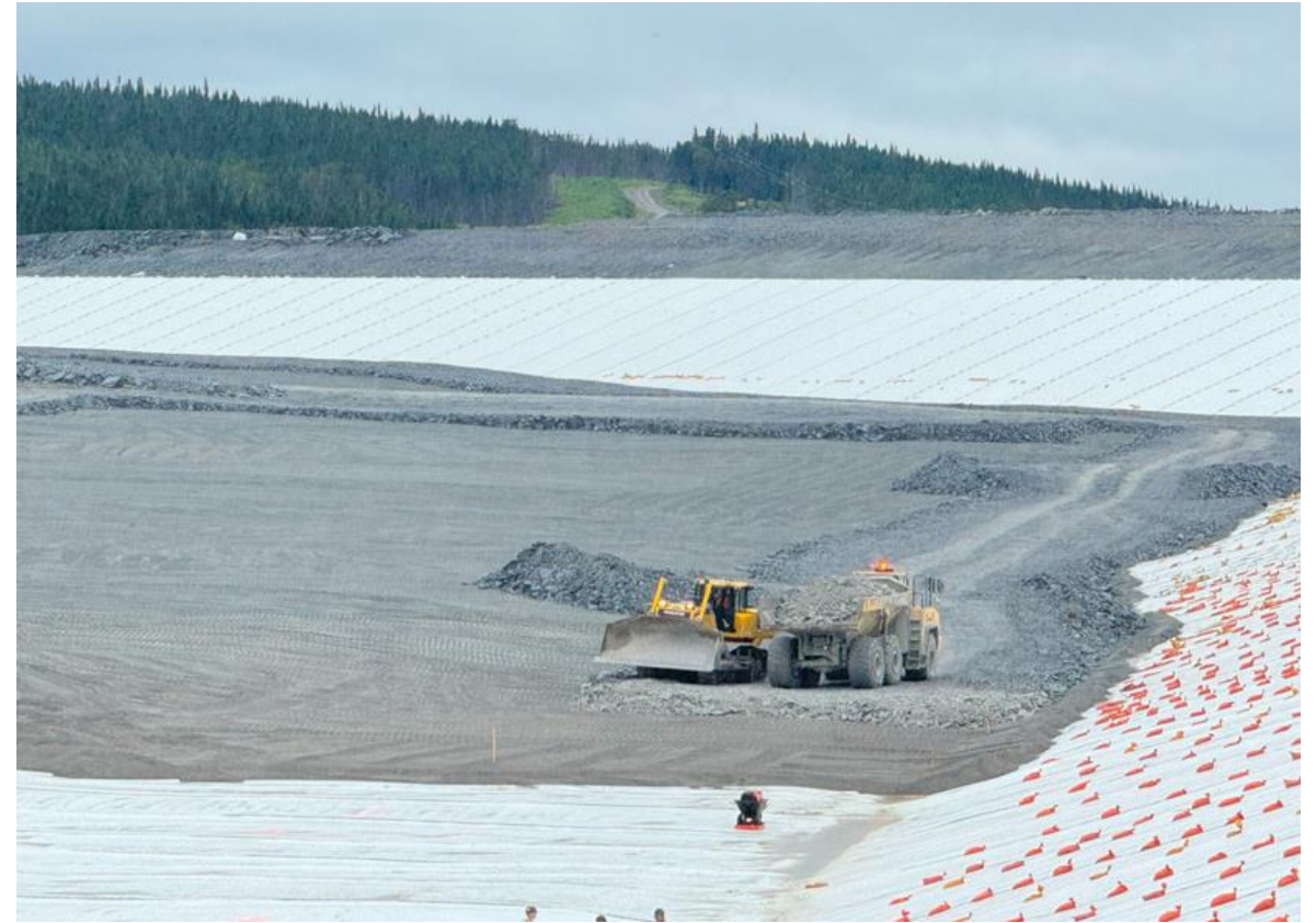
Tailings Management Facility Liner Progress
