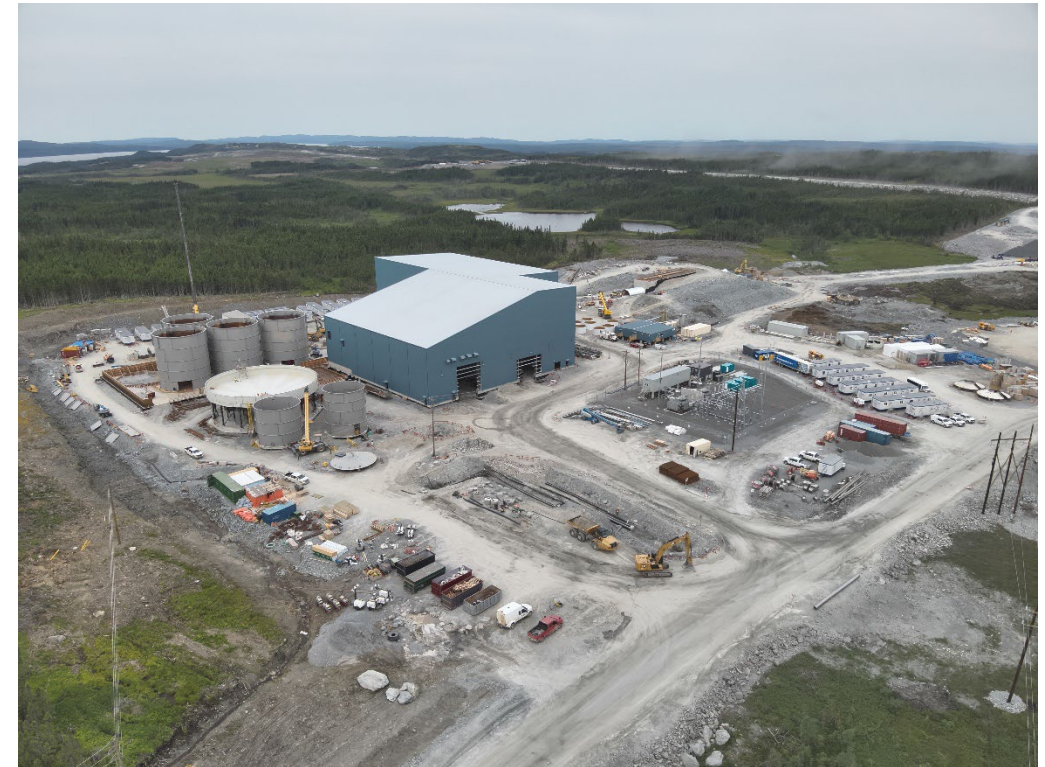
Valentine Gold Mine Plant Site (June 2024)
