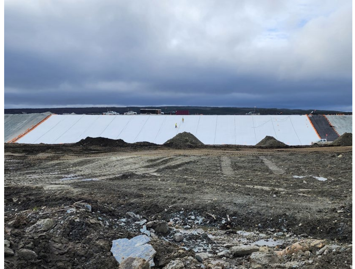
Tail Management Facility Liner Placement
