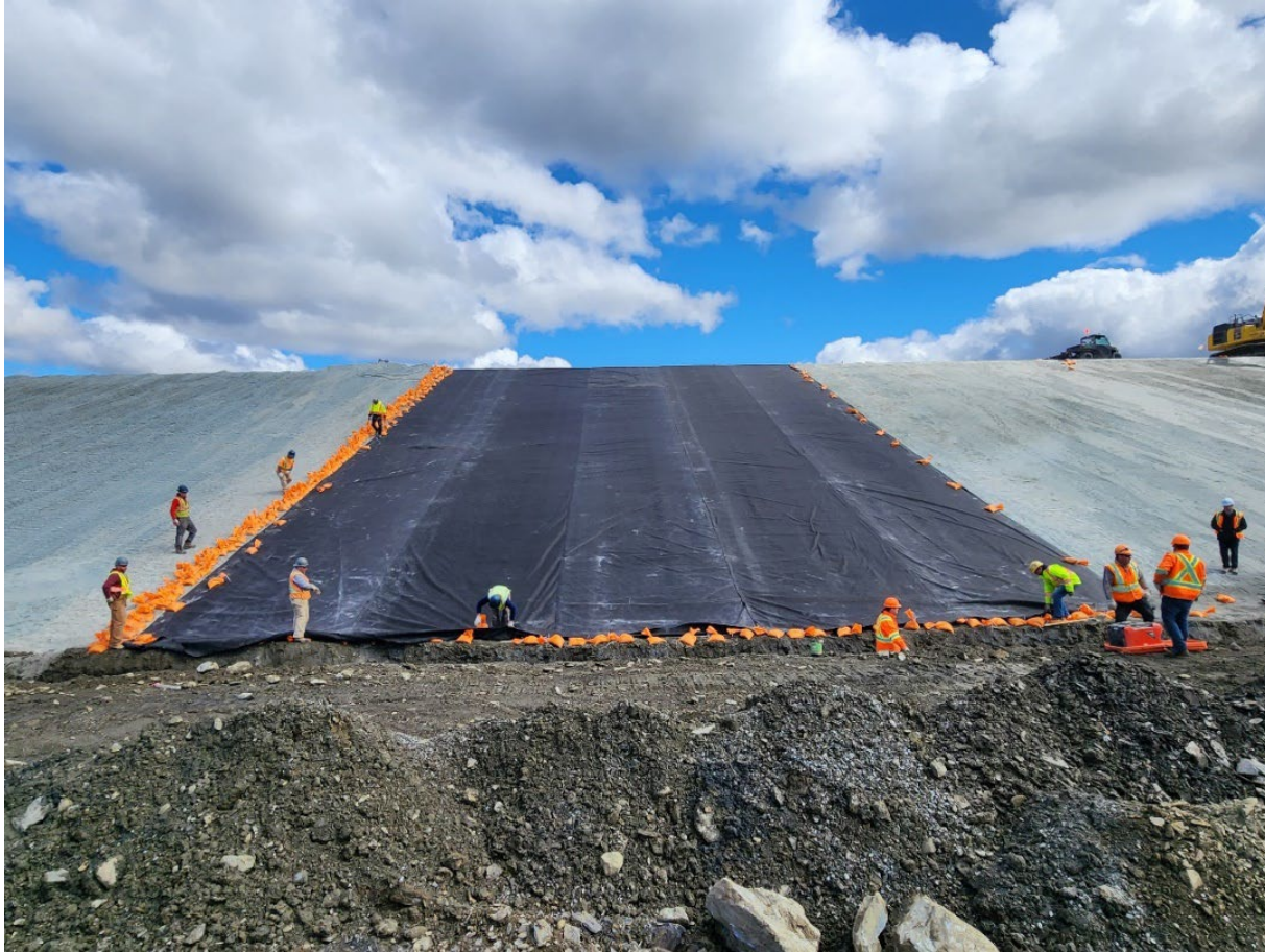
Tailing Management Facility Geotextile Placement
