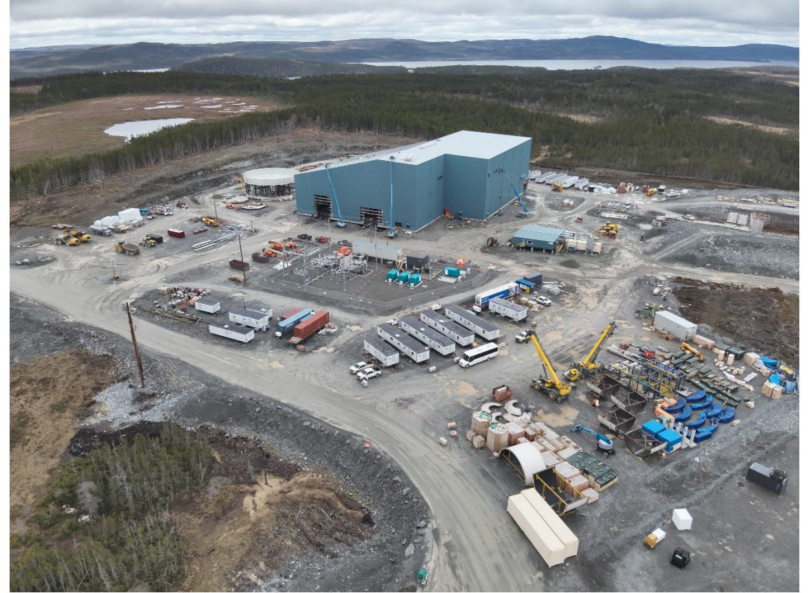
Process Plant Northeast
